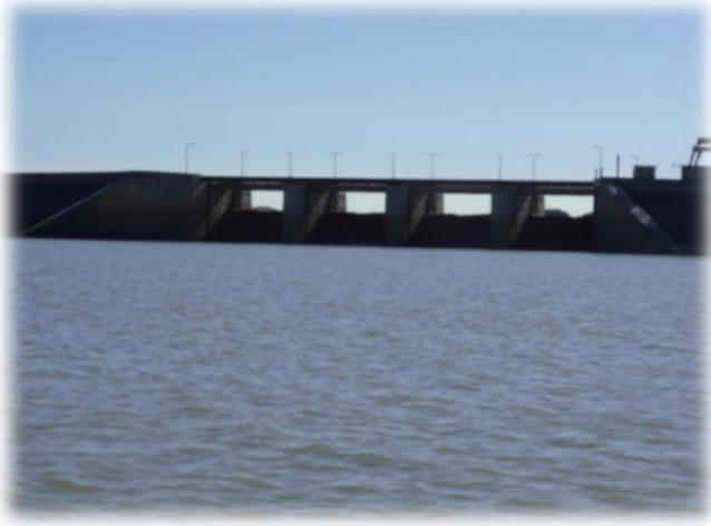
Hardap dam walls
